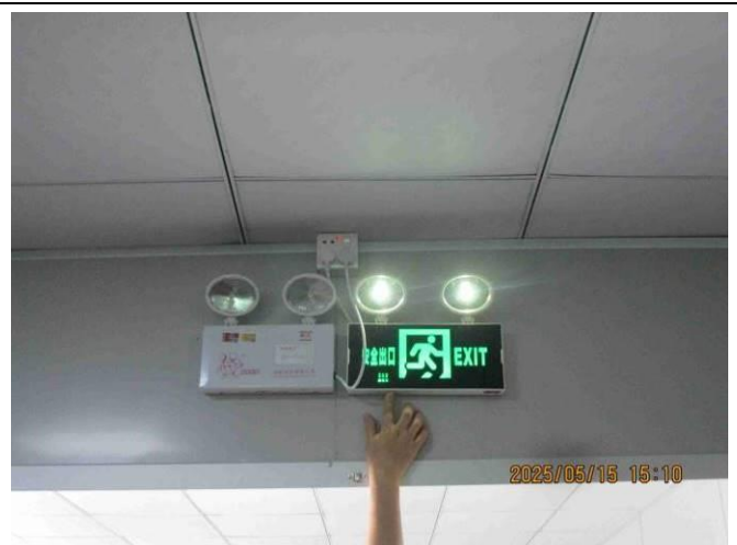
Emergency light testing
