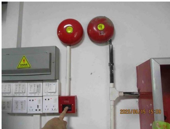
Fire alarm testing
