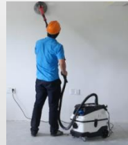
Tool work starts vacuum cleaner work immediately
