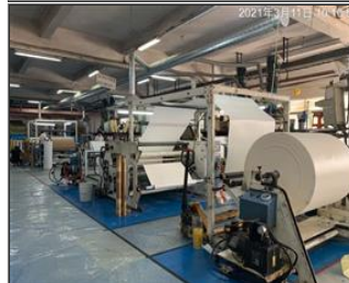
Photo of the inside of the main production hall Coating.JPG
