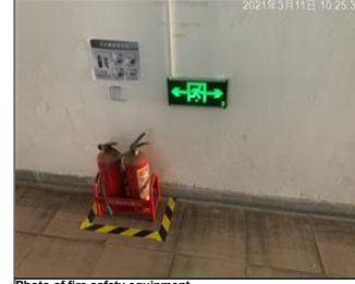
Photo of fire safety equipment Lampit evacuation indication sign 1 for dormitory building.JPG
