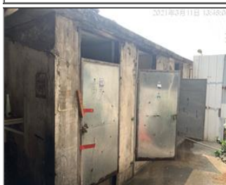
Photo of the sanitary facilities Toilet.JPG
