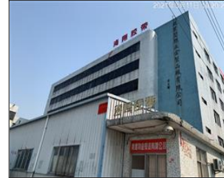
External photo(s) of the production unit(s) Production and warehouse building.JPG
