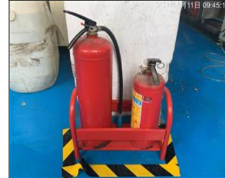
Photo of fire safety equipment Unblocked fire extinguishers and fire extinguishers were placed at the proper height 3.JPG
