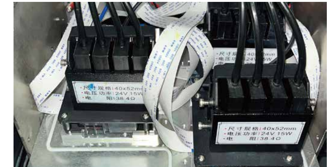
Base plate and damper heating
