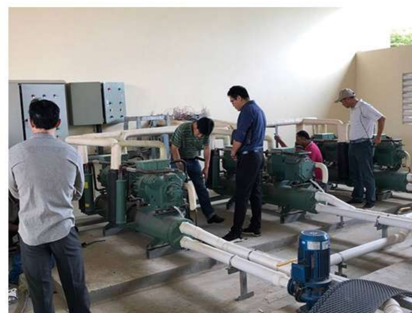
Compressor unit installation
