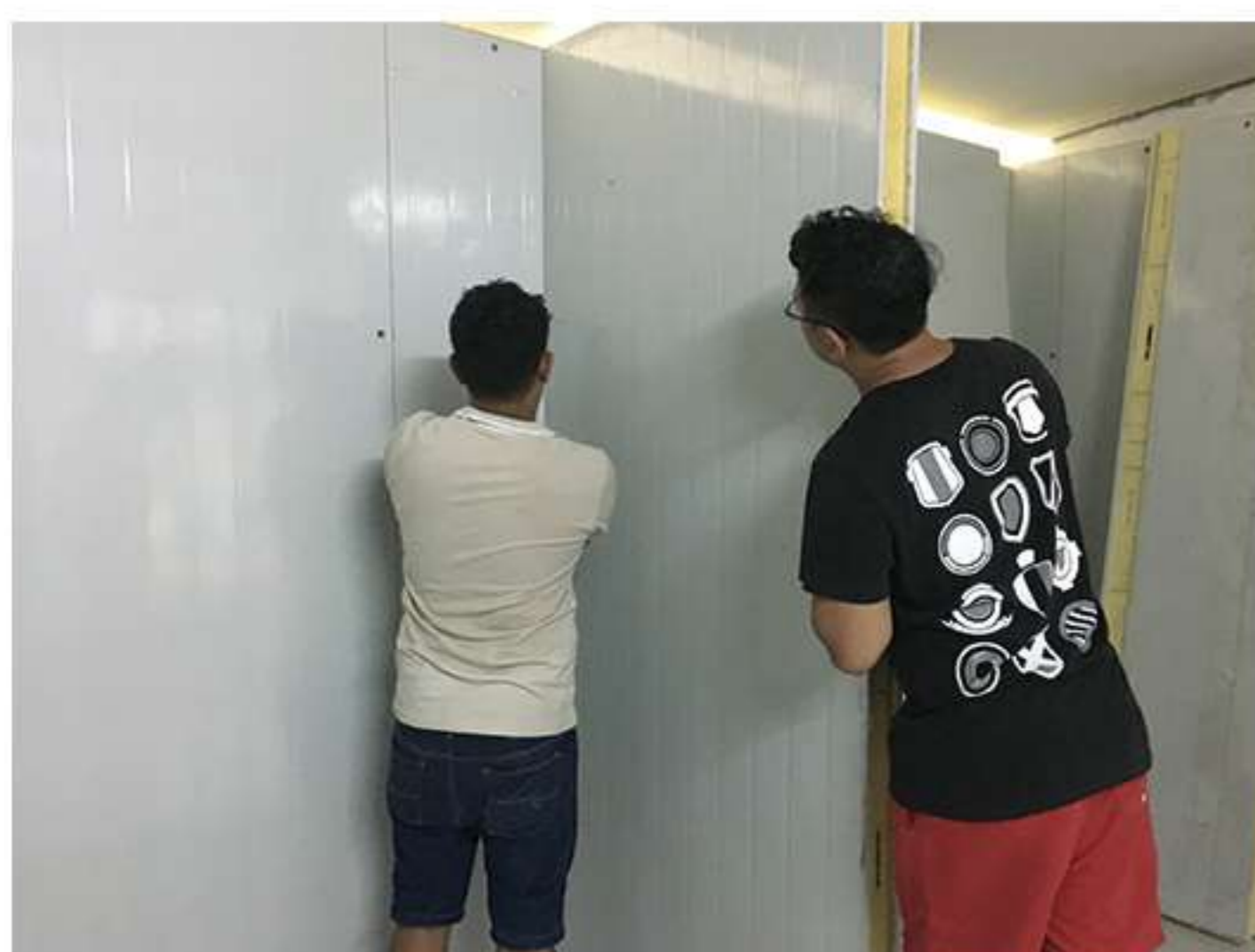
Cold room panels installation
