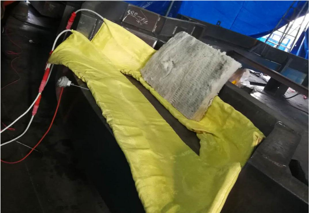
Preheating and post weld heat treatment for repair welding of thick walled castings
