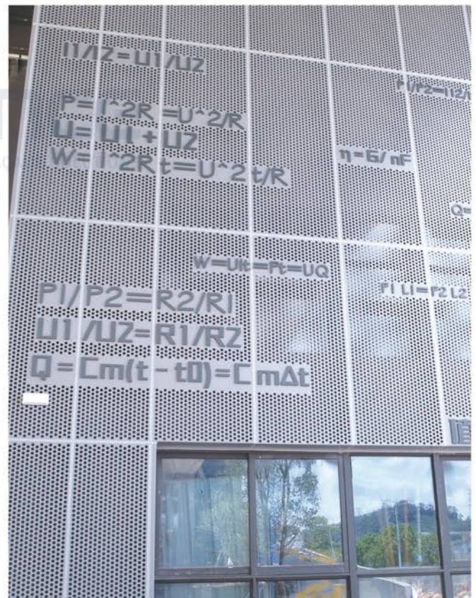
▲ The Project Uses a Punching Technique
