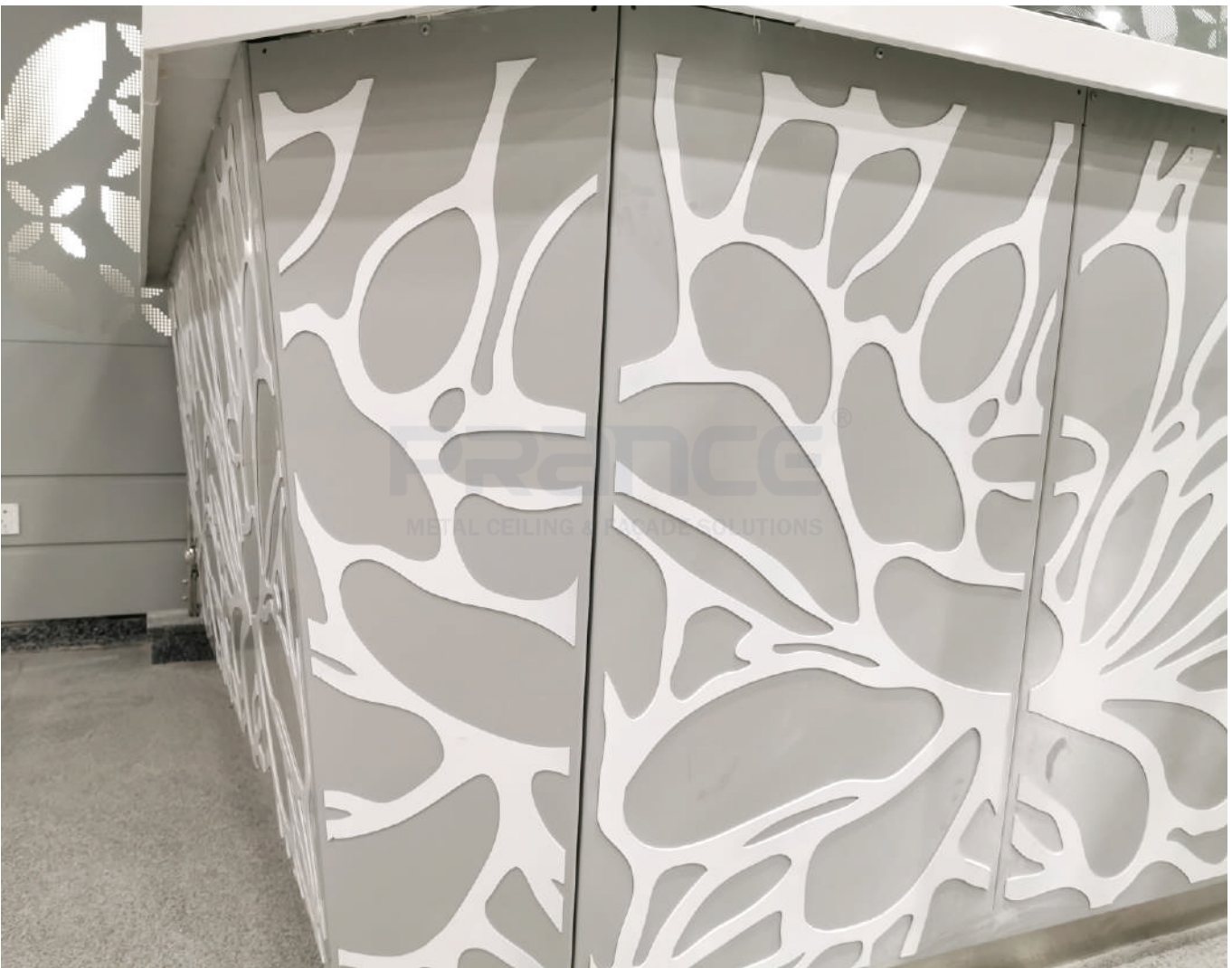
In this project, sculpted pattern aluminum panel assembly technology is employed for specific sections of the aluminum panels
