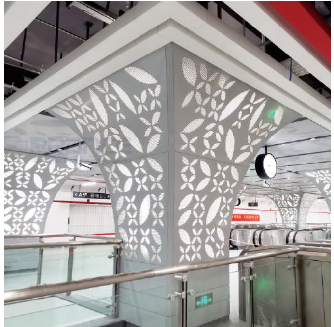
In this project, certain sections of the aluminum panels feature contour punching process technology
