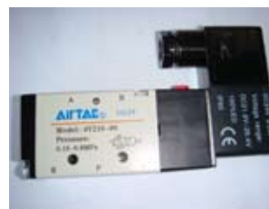
电磁阀 Solenoid valve
